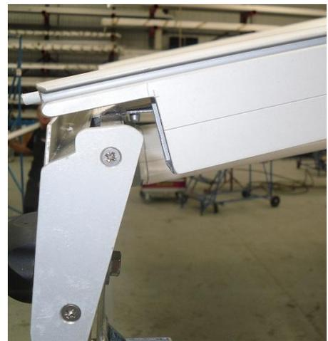
At the top of the rail you will notice a curved bracket, this locates onto the canopy lip. The cut out in the rail locates behind the fascia.
